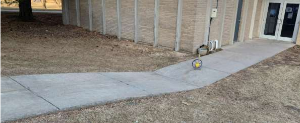
South East Ferguson Entrances Sidewalk, approximately 300 sq. ft.
