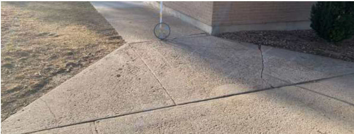
North West Library Sidewalk, approximately 200 sq. ft.
