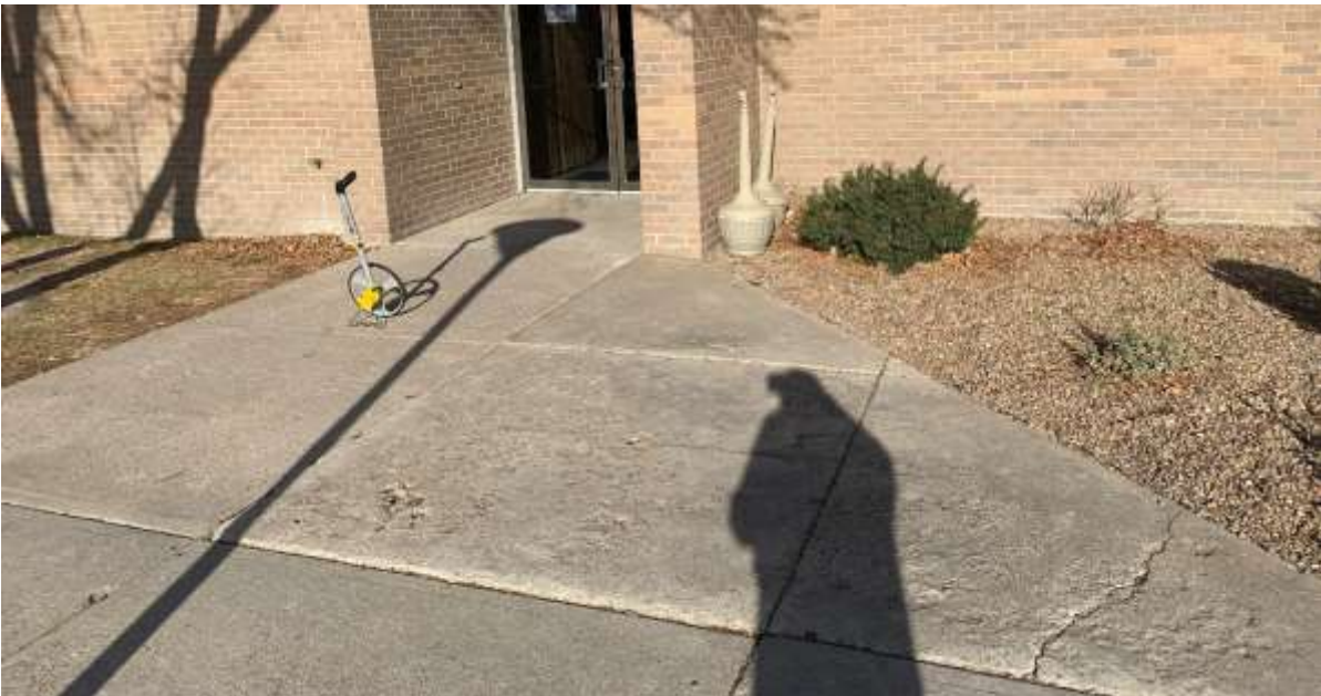
East Union Entrance, approximately 120 sq. ft.
