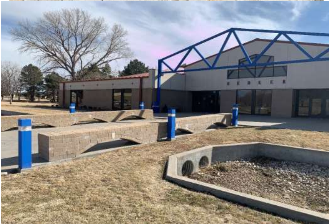
Bedker Hall Walkway Entrance. Total surface area, approximately 2,300 sq. ft.
