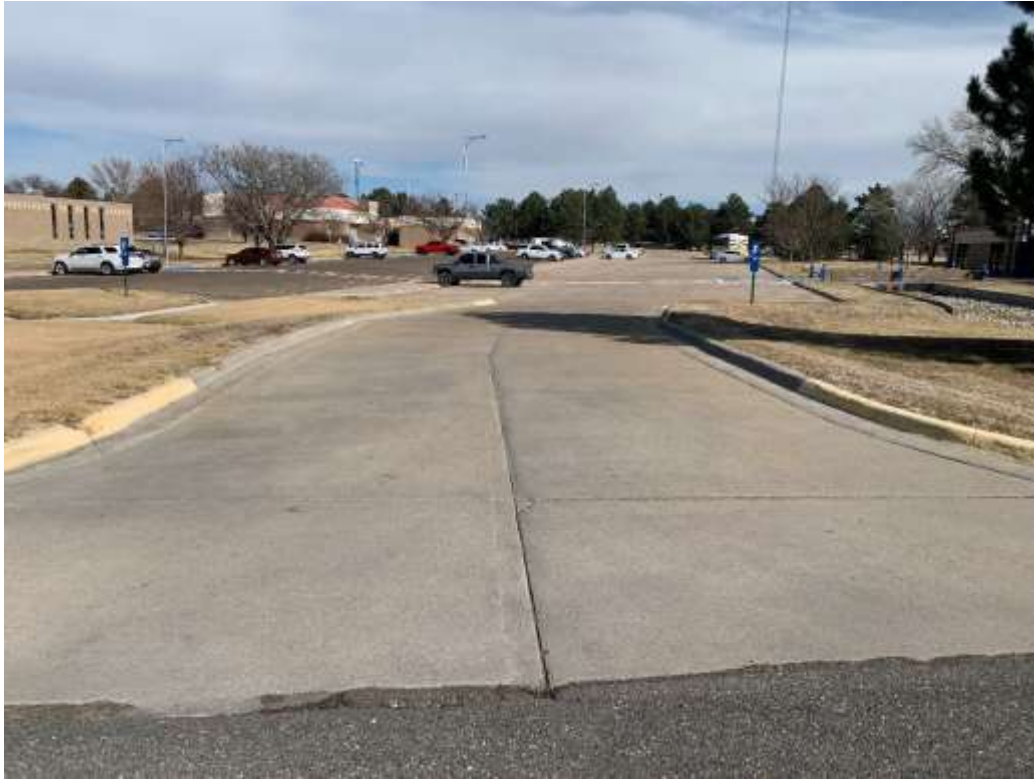
Entrance to Bedker Hall Parking Lot approximately 24' x 96'
