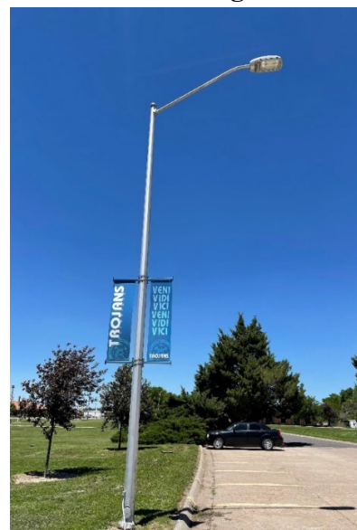
View Looking North
